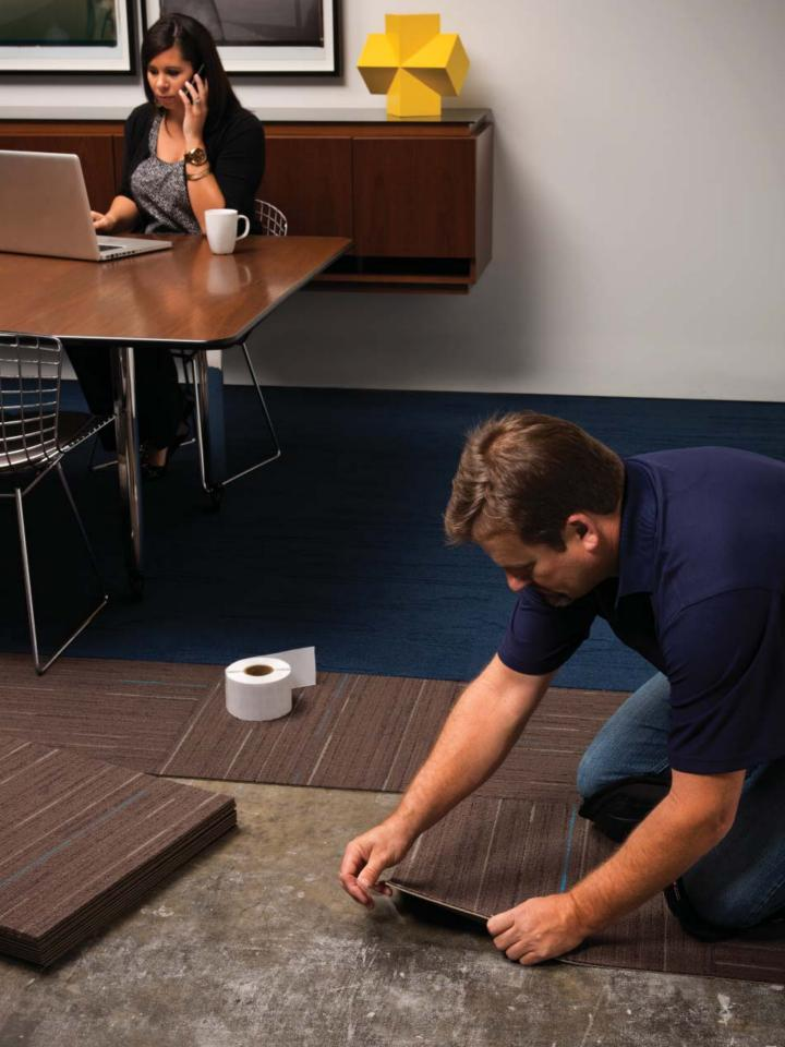
The mess and odor, along with the bulky containers and extra equipment associated with spread adhesives, only slow you down. Plus, you've also got to allow time for the glue to "set" before installing to prevent a cement-like adhesion that takes the flexibility out of modular carpet. While you're doing all of this, no one can work, play, shop, etc. because you can't have people and furniture in the way.
