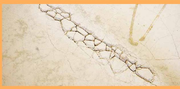
When you tear out stubborn, glue down broadloom carpet, sections of the subfloor, such as gypsum concrete, can adhere to the back of the flooring and cause much-needed repair before the next flooring installation. Upon repair, switching to a glue-free installation system eliminates this from future floor prep.
